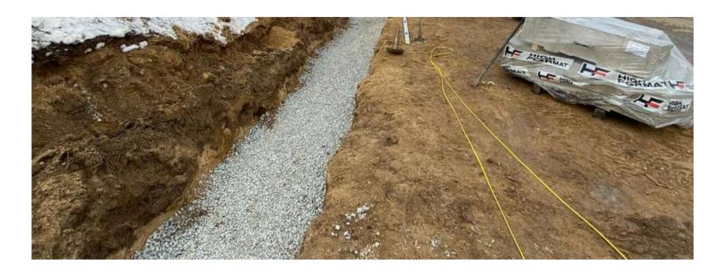
Proper base preparation is one of the most critical elements of retaining wall construction. The retaining wall is only as stable as the foundation it is placed on. If subgrade soils are deemed unstable or excessively soft, contact a qualified geotechnical engineer for remediation. The solution may entail over-excavating and replacing the soft soil with compacted granular material.
