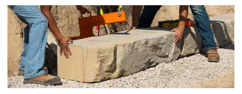
Proper placement of the bottom course of wall blocks is critical in determining the overall appearance and integrity of the finished project. Take extra time on this step and the rest of the project will go smoothly.
