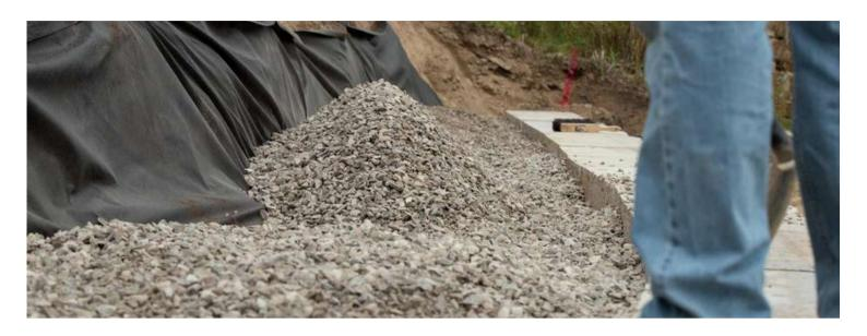
Appropriate selection and placement of backfill is necessary for the structural integrity of the wall. **Place only backfill materials which are consistent with the wall design.** For safety reasons, do not stack wall blocks more than 3 feet (0.9 meters) high before backfilling. **See Figure 2**.
