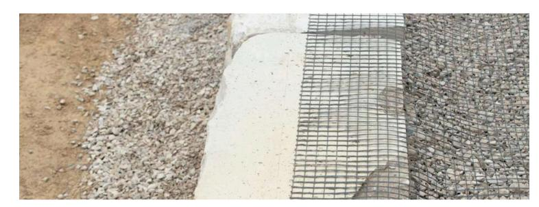
For walls that need to be taller than what is stable using an unreinforced, gravity-type structure (ie. stacked blocks), they can easily be reinforced with geogrid.
