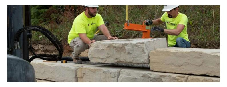
Placing the next course of blocks is similar to placing the first course. The primary difference is that you must engage the shear heels of the upper blocks with the backs of the lower blocks. Tips to accomplish this include:
